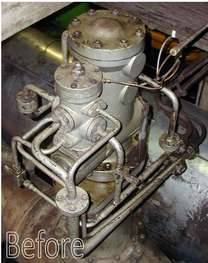
OLD CONSTRUCTION: Mechanical pilot control and complex pipework.
